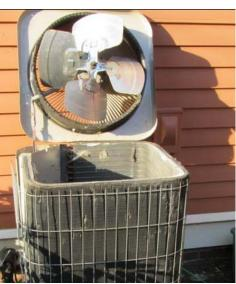
• **Observe** – If the equipment is no longer under water look around to determine how deep the water may have been. If the electrical components were not immersed the unit may only need cleaning. If the components have been immersed, replace them as even though they look dry internal damage may not be evident and chances are they will fail soon after when rust sets in.
