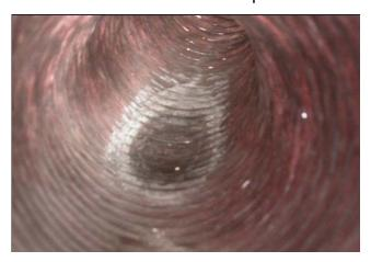
• **Diffusers and Grills** – Remove diffusers and grills to inspect the ducts beneath them. Rust, leftover mud and other debris can be another area where mold and mildew can begin to populate the duct system. Always inspect these areas to insure the heath of the occupants.
